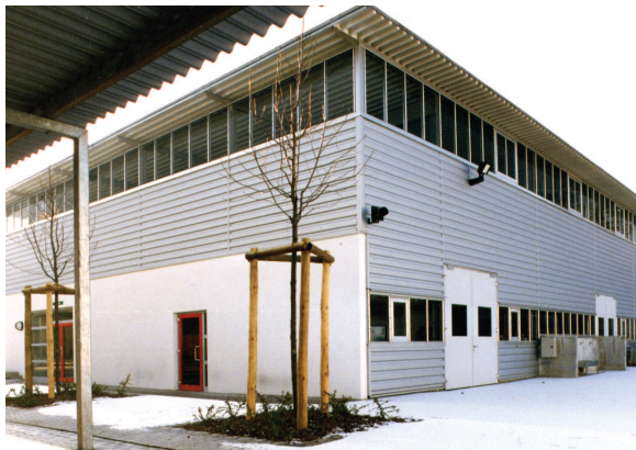
New building of an in-situ training yard
